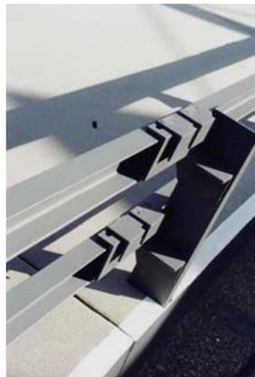
Fig.9. The first trestles and deck units including crash barriers are installed
