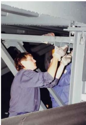
Fig.8. Simple bolt connections for securing elements
