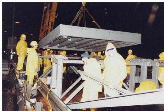
Fig.7. The first flyover deck unit is placed on the trestles arranged symmetrically on either side of the expansion joint
