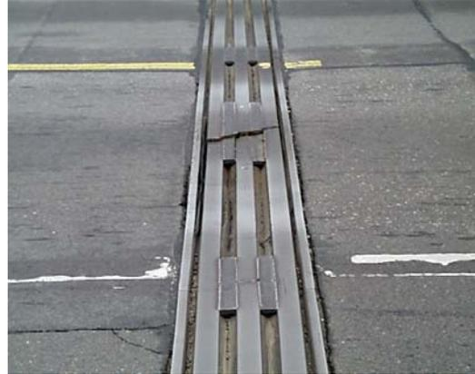
Fig.6. Makeshift repair of Expansion Joint
