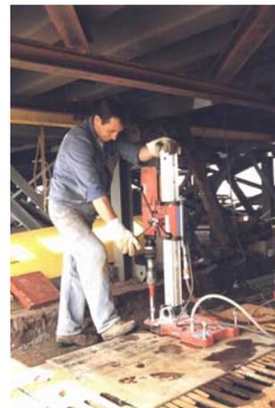
Fig.2. The exchange of an expansion joint underneath the ramp
