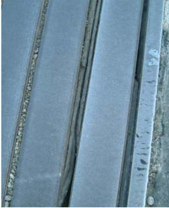
Fig.5. The rubber profiles and the small stones blocking the sealants and membranes
