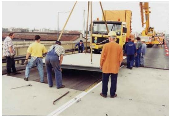
Fig.11. The last flyover deck unit is positioned.
