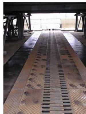
Fig.4. The new finger expansion joint [1]
